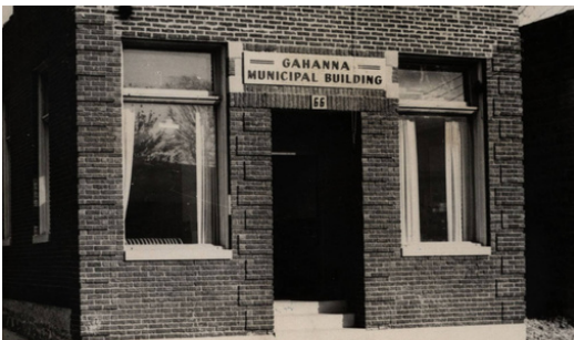
The Gahanna Bank/Municipal Building
