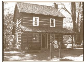
Notice the architectural detail of the Log House! You will see that the builders added a great detail to keep water out, a drip ledge. In addition, this log house (not to be confused with a log cabin) was built using dove tail construction, a specific type of jointing. This home is a log house and not a log cabin because it is two stories, and the logs are hewn.
